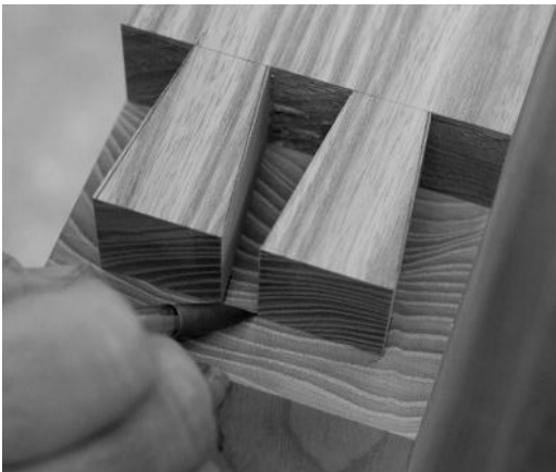
Marking the pin locations from the tails.
